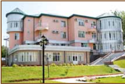
Training and Health Centre of the National Bank of Tajikistan (Kayrakkum)
