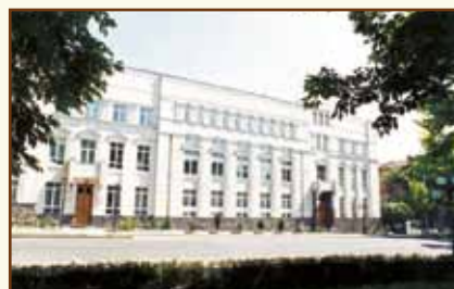
Central Bank of the Republic of Armenia Administrative building
