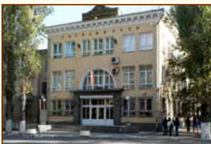
National Bank of the Republic of Kyrgyzstan Administrative building
