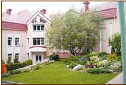
The Training Centre of the National Bank of the Republic of Belarus (village of Raubichi)
